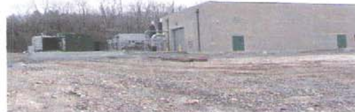
The Fitchburg Landfill Gas to Energy Project
