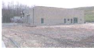
The Fitchburg Energy Project- See page 2 for more information
